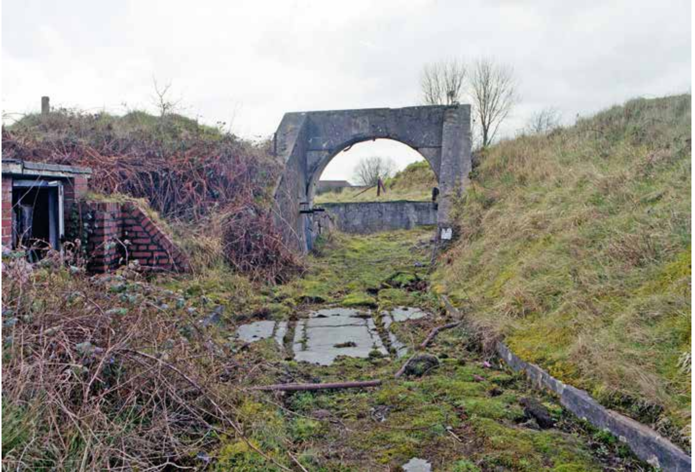
The 'Jamaican Tar' trolley route to the nitrating houses in 2002. The trolleys were manually pushed full of Nitro Glycerine. The Jamaican tar was used as it was renowned to be very spark resistant. This area forms part of Nitro Glycerine Hill which has now been made a Scheduled Ancient Monument by CADW. Photo Nick Catford
